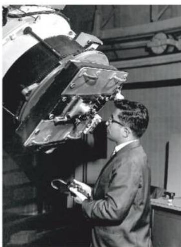
USNO astronomer Mihran Miranian centers a target in the photographic double star camera prior to installing the photographic plate and beginning a series of observations, in this picture taken in the mid-1970s. USNO LIBRARY
