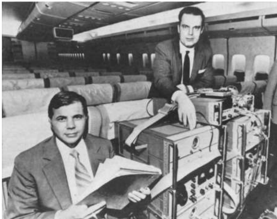
Joseph Hafele (left), Richard Keating, and their HP-5061A cesium clocks prepare for one of their two round-the-world flights, October 1971
