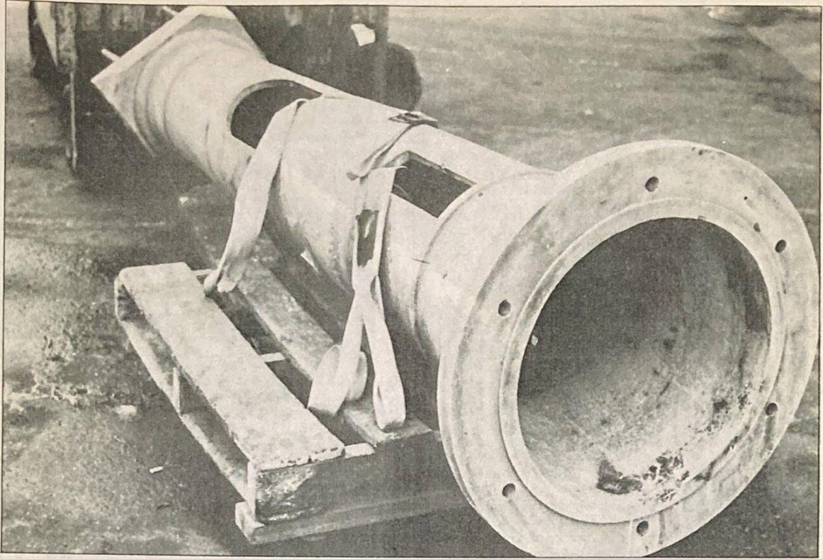
*The largest parts of the telescope were taken to a local company for chemical derusting and paint stripping. The cast iron pier, pictured here, came out looking like new.*
