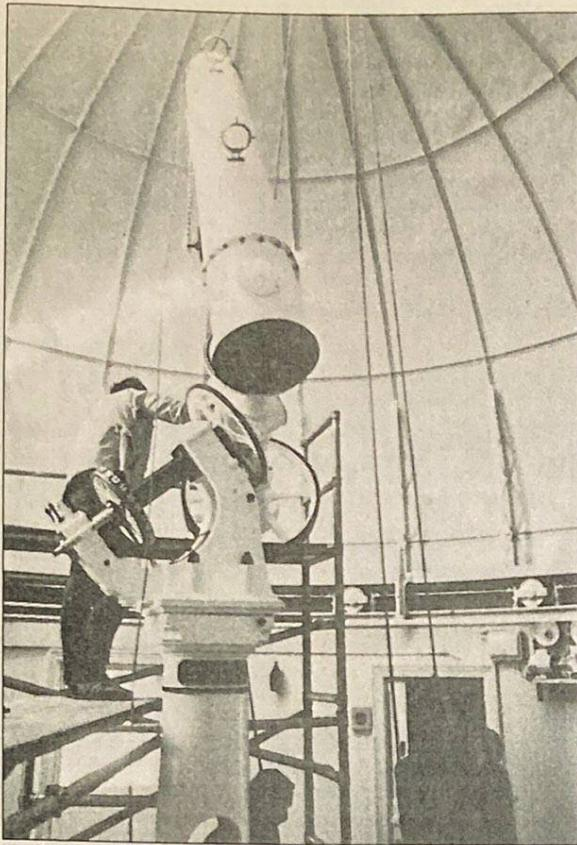
*Assembling the tube of the telescope proved difficult since as each section was installed, the balance of the instrument would change dramatically. A scaffolding was used to support the counterweight of the declination axis while ropes held the tube sections.*
