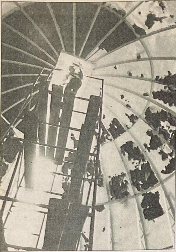
*Before the telescope was installed, the interior of the dome had to be cleaned and painted. Rich Schmidt is shown blasting old paint off the dome using a high-pressure air hose.*
